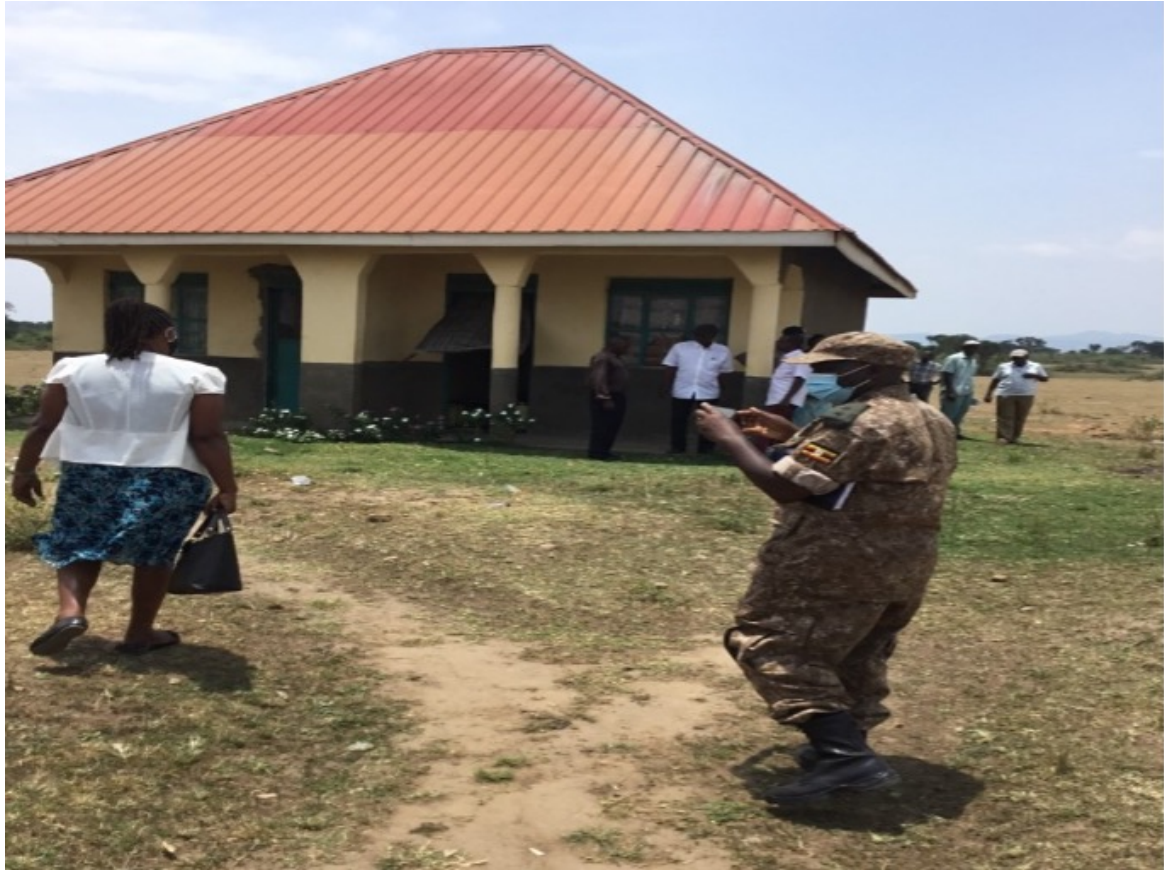
A Staff quarters constructed at Hamukungu Primary School Queen Elizabeth National Park
